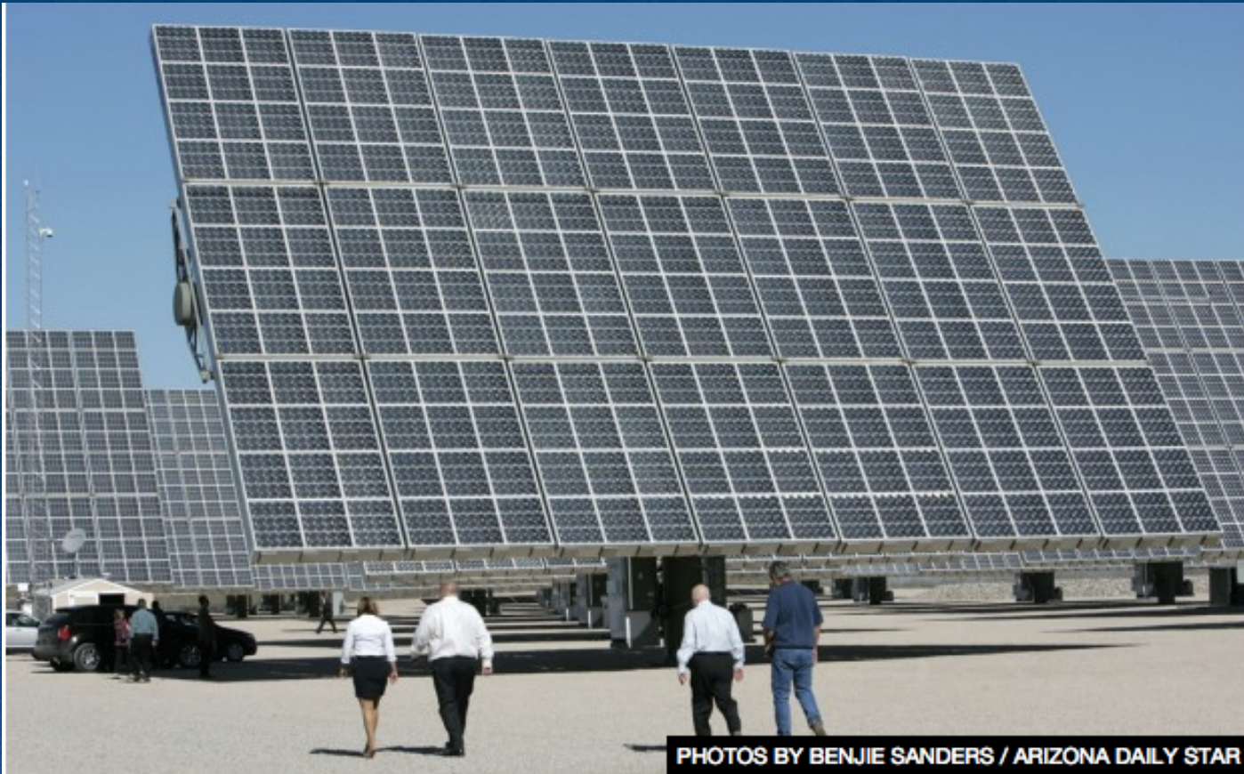
A new 12-acre solar-energy system at UA's tech park features 36 huge solar panels, each about the size of an IMAX movie screen.
